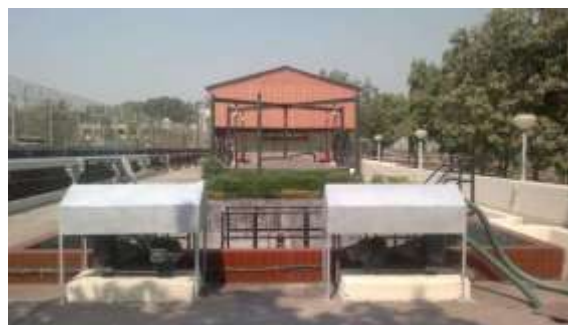
Bird's Eye view of the Bio Gas Plant
