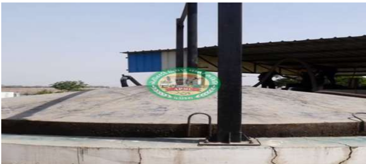
Fig-3 Green Waste (duly crushed) added to Gas Chamber
