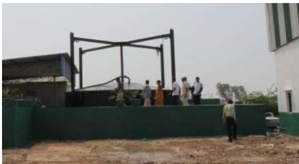
Gas holder with lifting arrangement and Gas Pipe
