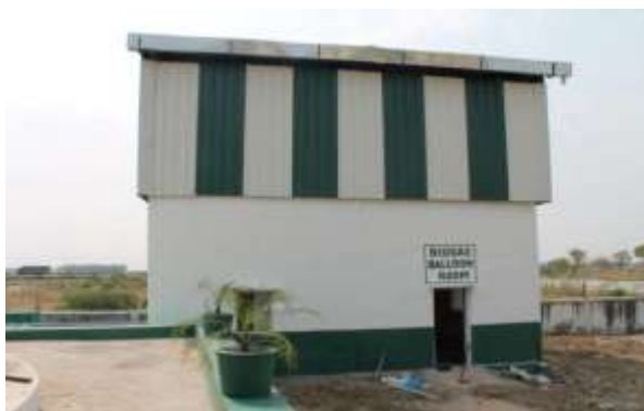
Room for storing excess Gas Balloon
